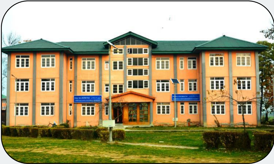
ECE Department Building
